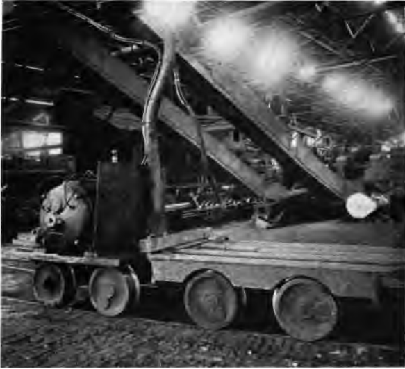
The Motor-Driven Bloom Carriage
